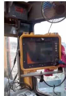
Fig 1.1. Typical on-board rig computer
