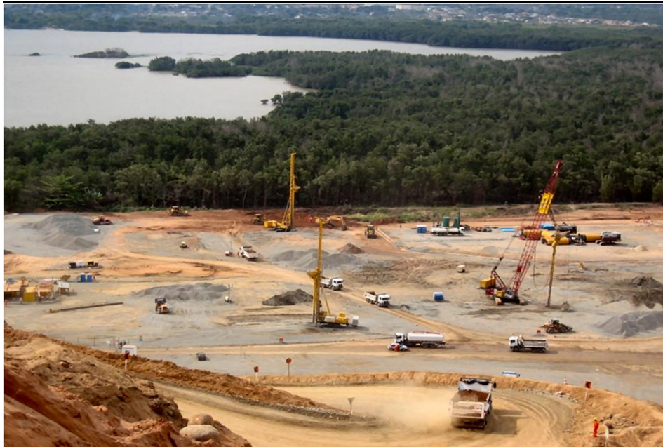
Ground improvement for iron ore stockyard facility
