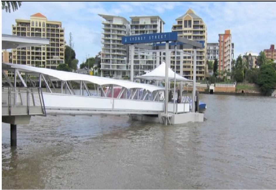
Ferry terminal reconstruction
