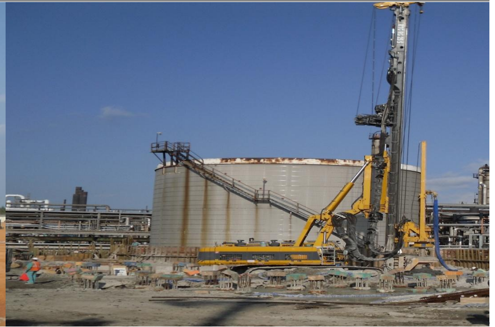
CFA piling at oil refinery
