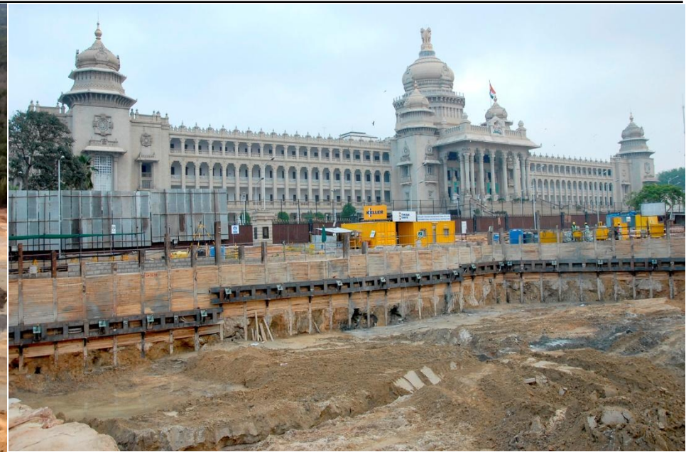
Anchors for new metro
