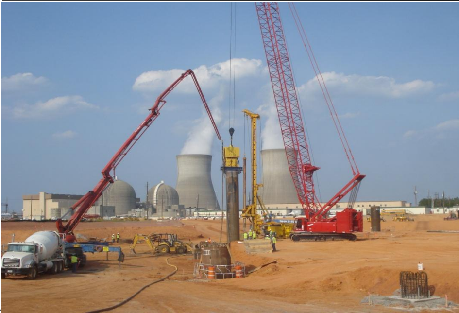
Bored piling at nuclear power plant
