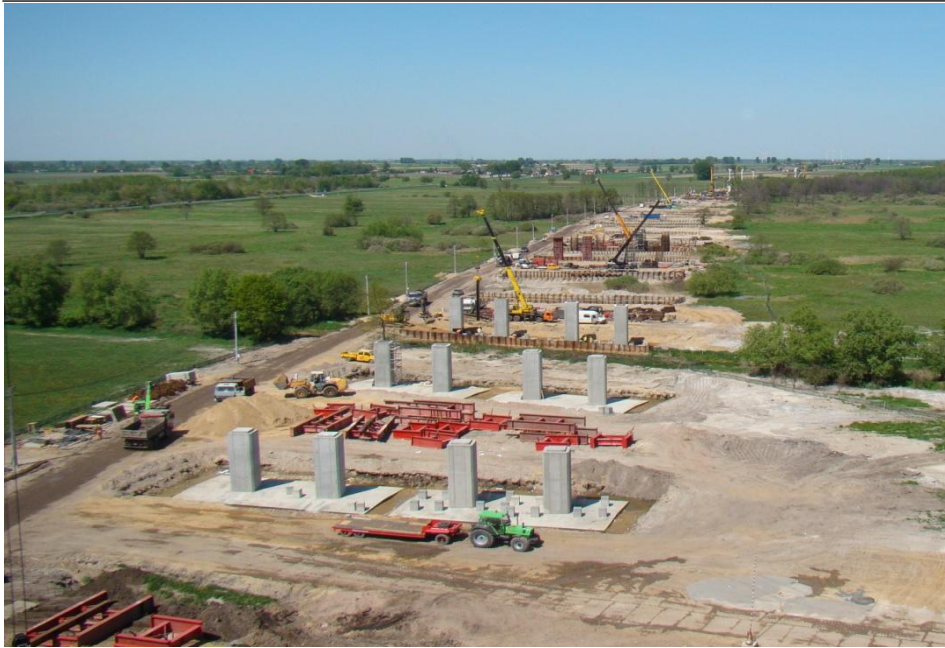
Bored piling for bridge
