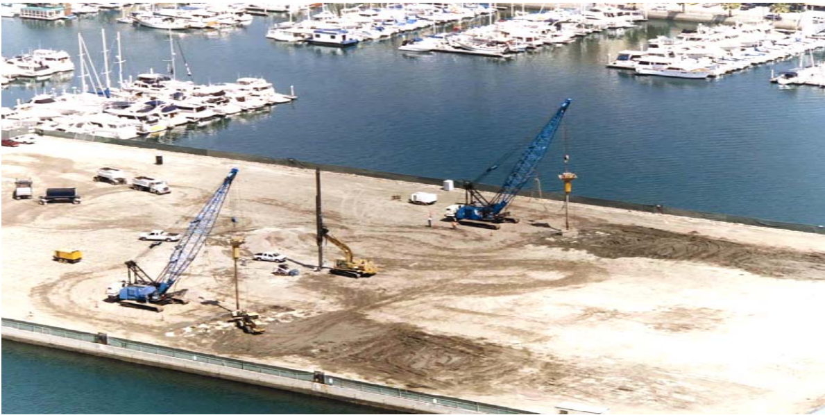
Hayward Baker Soil Mixing & Vibro Replacement Waterfront Condominium Development Los Angeles
