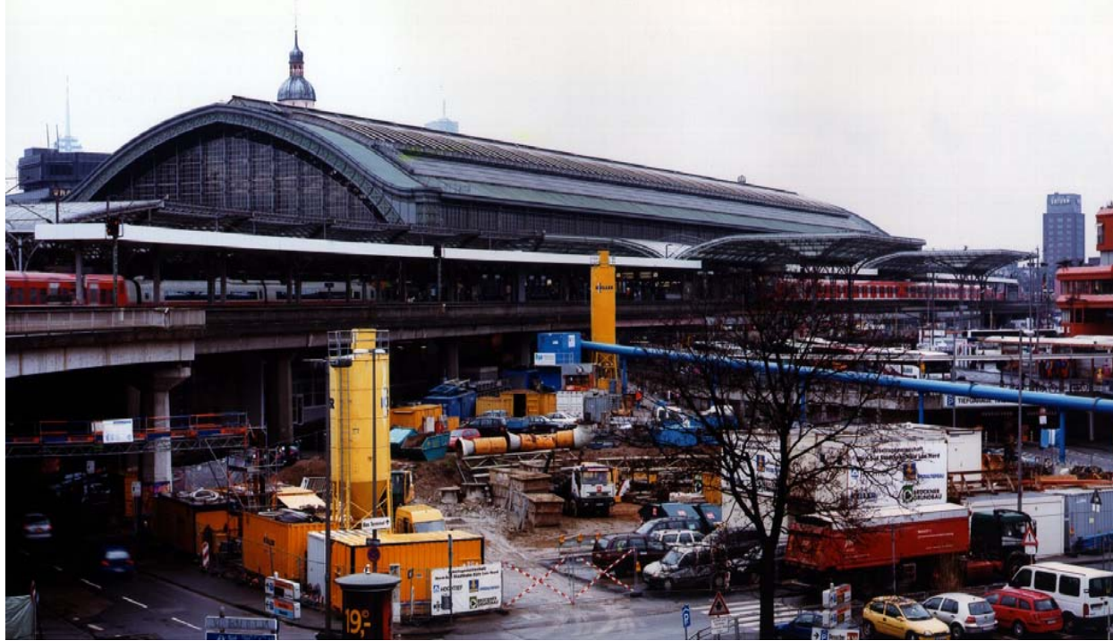
Germany Grouting and Anchors New underground rail link, Cologne
