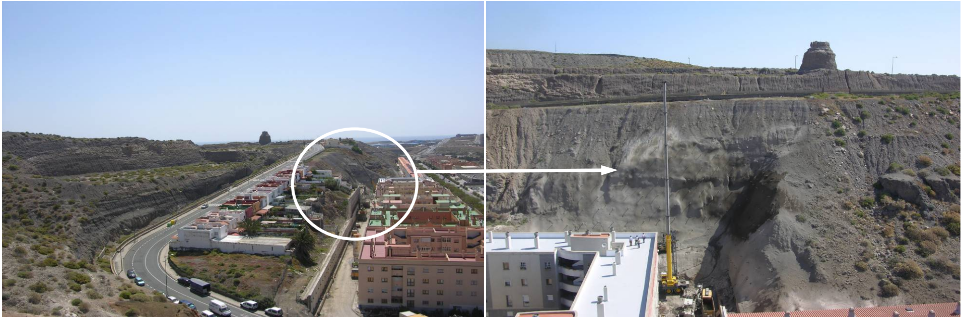
Site of emergency works
