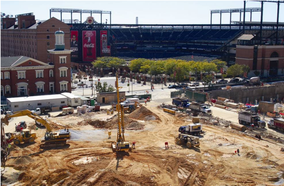
Hayward Baker Baltimore Convention Center Design build contract Vibro piers
