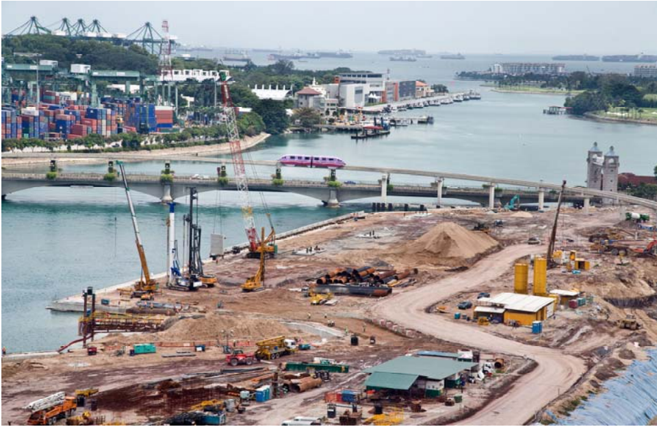
Sentosa Island, Singapore New resort complex Wet soil mixing
