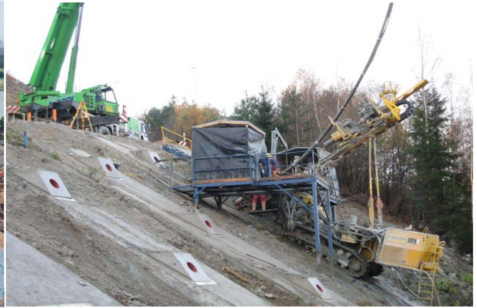
A2 Motorway, Austria Slope protection Anchors
