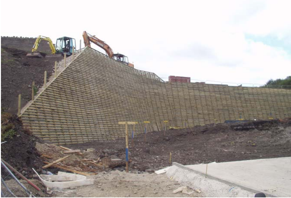
New supermarket, Maesteg, Wales Retaining permacrib wall Phi
