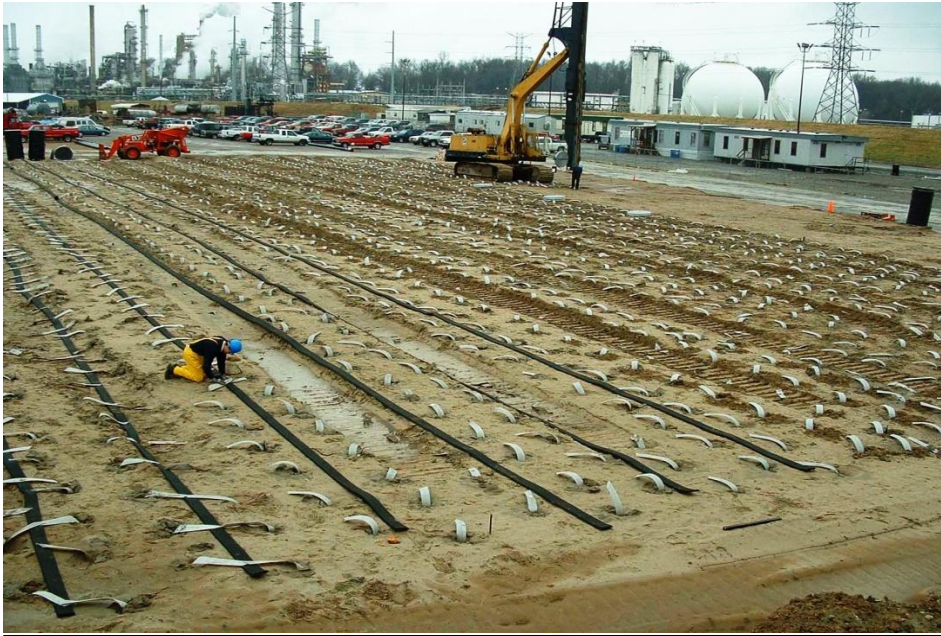
Nilex installing wick & strip drains
