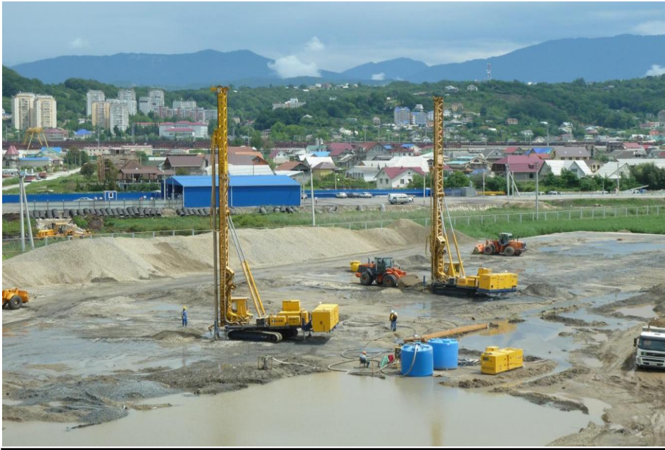
Vibro compaction and jet grouting 2014 Olympic Park, Sochi, Russia
