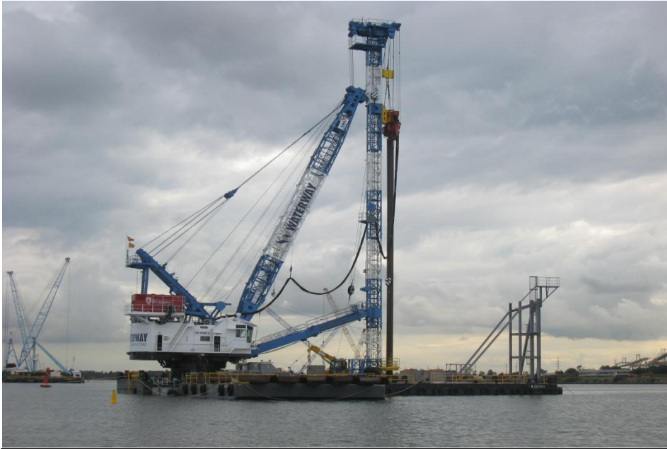
Installation of sheet pile wall Hunter River, Newcastle, NSW
