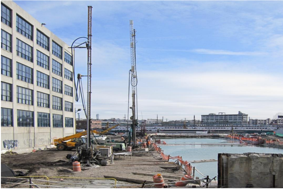
Jet grouting for new rail tunnels Borough of Queens, New York
