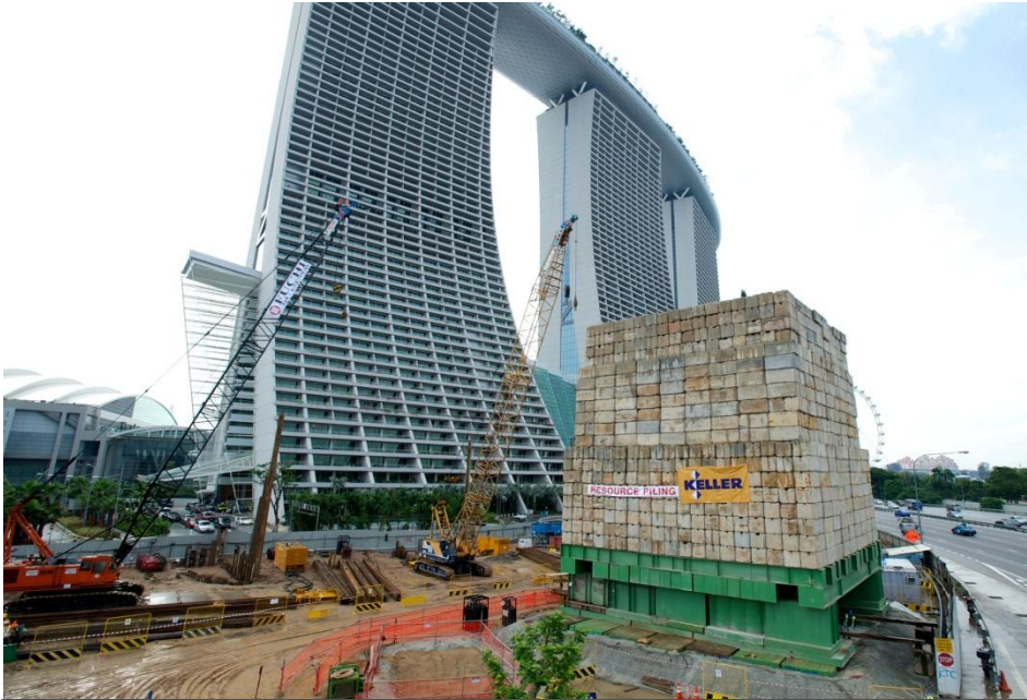
5,700 Ton Load Test Marina Bay, Singapore
