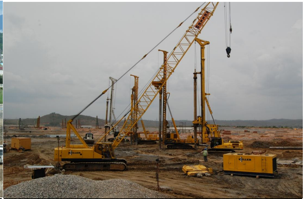
Vibro replacement and bored piling Power plant, Anpara, Northern India
