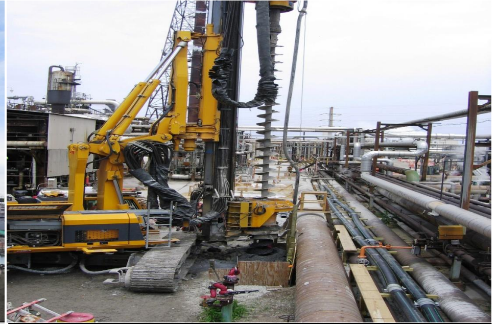
Piling at oil refinery Whiting, Indiana
