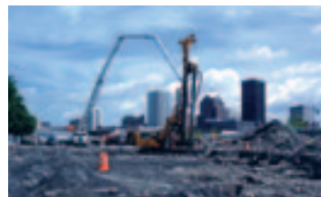
Hayward Baker installs vibrated concrete columns at the Corn Hill Landing Buildings, New York State, USA.
