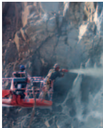
Hayward Baker undertakes slope stabilisation works for a luxury villa construction on Peter Island, British Virgin Islands.
