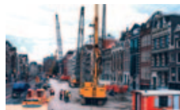
Keller Grundbau performs jet grouting at stations on the Amsterdam Metro, Netherlands.
