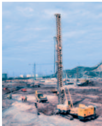
Keller-Terra undertakes ground improvement with stone columns for a combined cycle power plant in Murcia, Spain.
