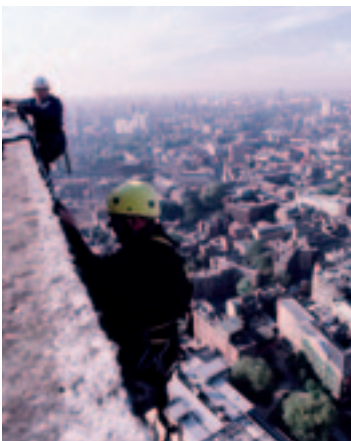
Makers uses abseil access to carry out a concrete condition survey at Trellick Tower, London, England.
