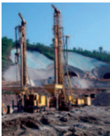
Geotechnik undertakes ground improvement works for a new motorway at Krapina, Croatia.
