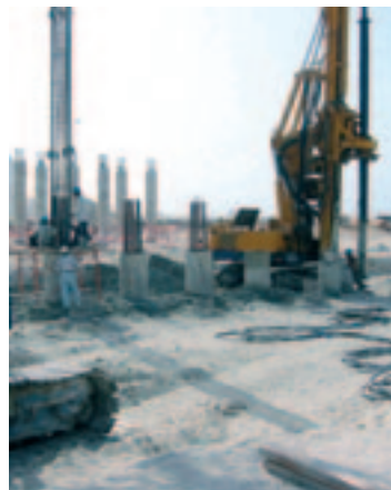
Keller Grundbau installs bored piles to support two new road flyovers at the North Manama Corridor, Bahrain.
