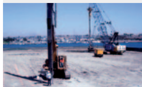
Hayward Baker undertakes soil mixing and vibro replacement works for a waterfront condominium development at Marina del Rey, Los Angeles, USA.
