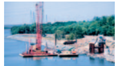
Case installs drilled shafts to support a bridge over the Tennessee River in Kentucky, USA.
