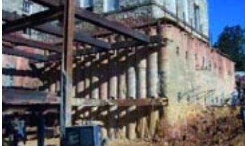
McKinney constructs a secant pile wall for the University of Virginia, US.
