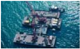
Case installs four water intake shafts for a new power station at Lake Michigan, Wisconsin, US.
