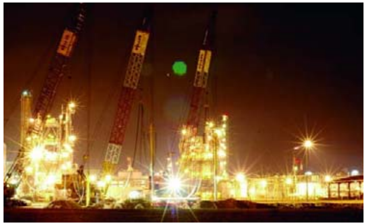
Keller Singapore operates up to 12 vibrators around the clock to complete vibro compaction works for a land reclamation project in Jurong, Singapore.
