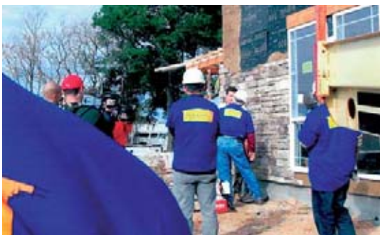
The Suncoast team involved in providing foundations for a new home for a disadvantaged family in Houston, Texas, US.
