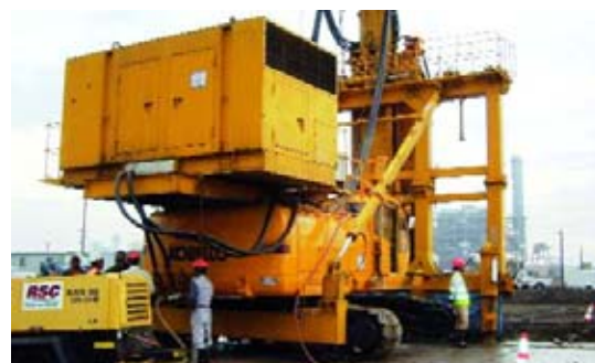
Hayward Baker tests the new "TRD" equipment used for trench cutting and installation of barrier walls at Los Alamitos, California, US.
