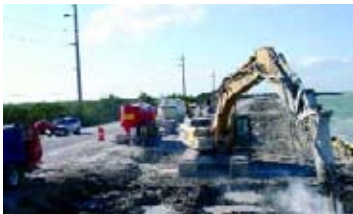
Hayward Baker uses soil mixing to strengthen the ground for a road widening scheme in Florida, US.
