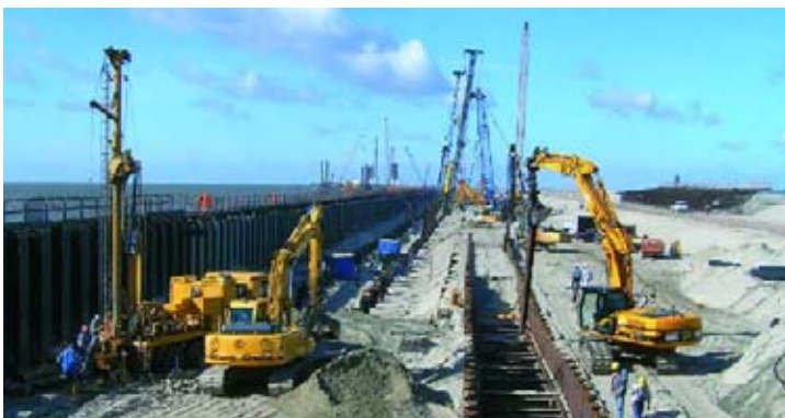
Keller Grundbau and Keller GeTec undertake site investigation and monitoring works for the construction of a new container terminal at Bremerhaven, Germany.
