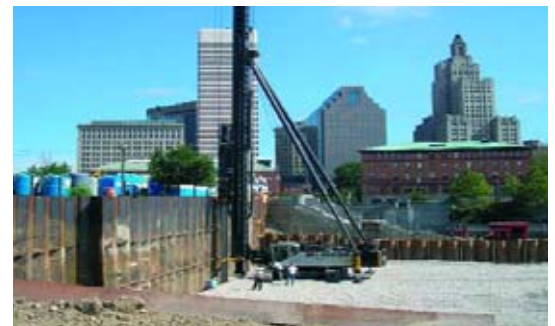
Donaldson installs steel sheet piling and precast piles for a 23-storey mixed use building in Providence, Rhode Island, US.
