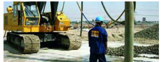
KGE provides a "package solution" including earthworks, remediation, dynamic compaction, piling and vibro techniques for a regional housebuilder at Rainham in Kent, UK.
