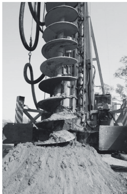
Top Drilling of bored piles at a residential development in Pymble, a suburb of Sydney.
