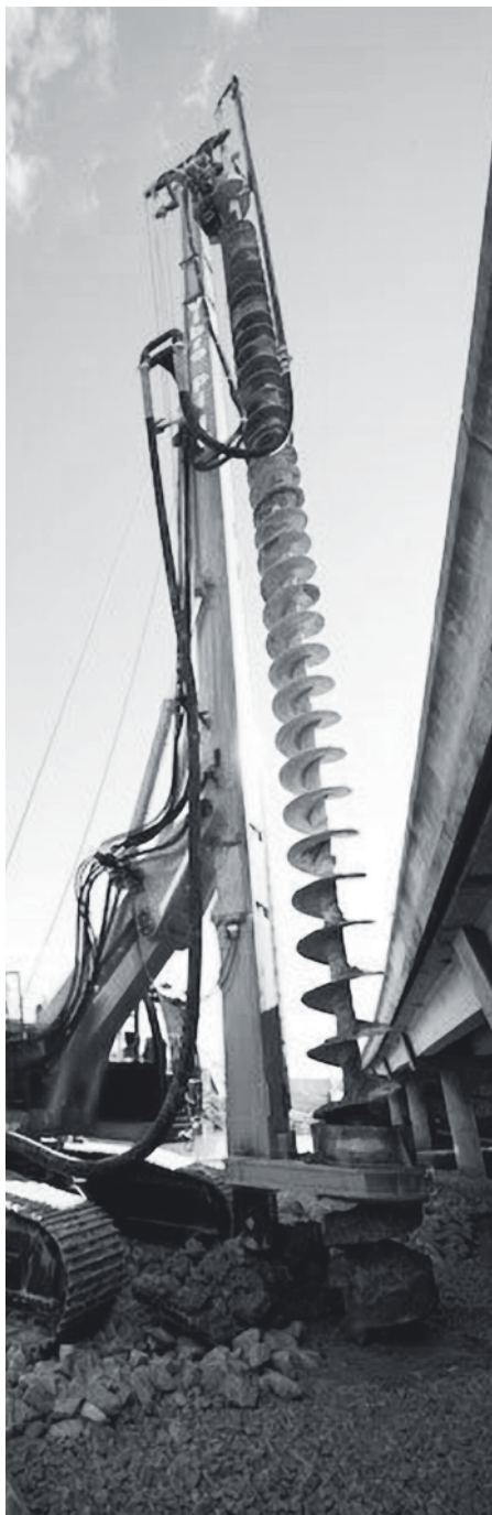
Above Continuous flight auger piling for the Monash Freeway upgrade at Dandenong Creek Bridge, Victoria.
