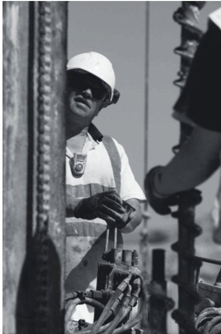
Top Installation of tension piles, removable ground anchors and a grout curtain for the SouthGate centre in Bristol.
