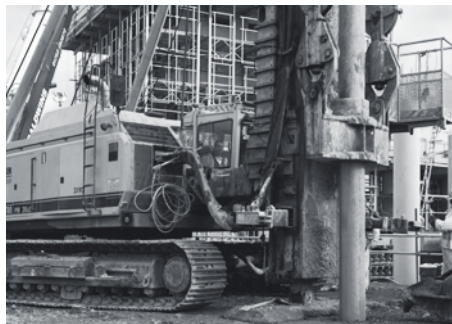
Above and right Installation of driven cast in situ piles, continuous flight auger piles and vibro concrete columns for the 2012 Olympics Stadium in London.
