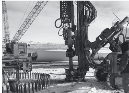
Above Construction of foundations for a wind farm in Mountain Home, Idaho.
